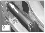
Position the mount shaft and channel inside the door as shown to determine the shaft location.
