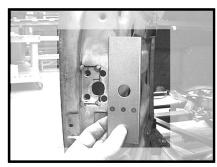
8) Now position the latch plate behind your drilled area and weld in place.
