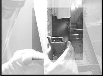
3) Cut out area. Make sure you have access to install the latch from the back.
